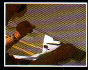
STEP 2: Position a strip of masking tape 1/2-inch from the bottom of the transom along the entire mounting surface.
